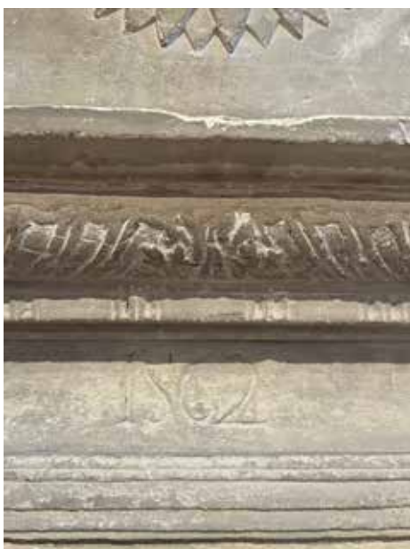
Fig 8 Detail of the Chaldon tablet showing the inscribed date 1562, multiple forms of mouldings and decoration, plus remnants of paint/applied surface decoration in pattern carved into the ovolo moulding midway between the date and the sun
