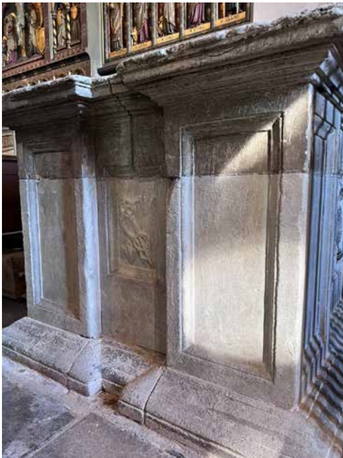
Fig 3 Cawarden tomb, Bletchingley seen from the south-west. Note the relative simplicity of the mouldings and the contrasting tones of the stone used.
