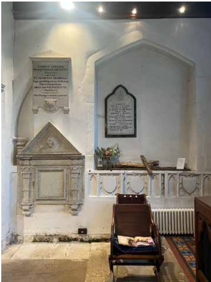
Fig 2 The north wall of the chancel, showing location of tablet relative to blocked arch and blocked window aperture (this and all subsequent photos by Rob Briggs)
