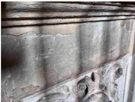
Fig 7 Remains of paint or other surface-covering layer on south side of the Cawarden tomb
