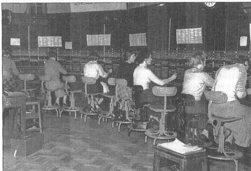
Fig. 7 A view of part of the manual switch-room at Redhill manual exchange in the late 1950s. Incoming calls appeared on the lower part of each board's fascia, and outgoing calls to other exchanges were connected via junctions on the mid part of the fascia. The multiple of all Redhill numbers can be seen at operators' head level above these, with plenty of room to grow vertically.
