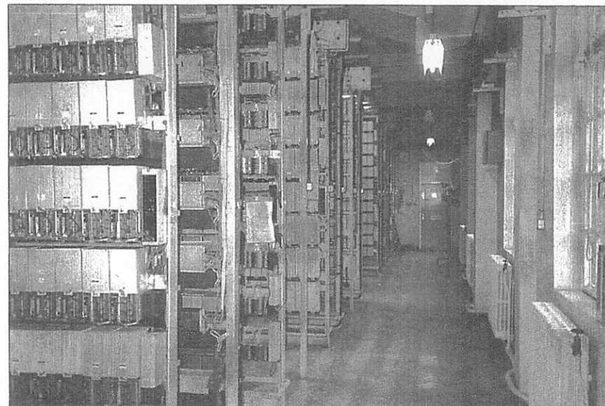
Fig. 10 A small part of the first-floor apparatus room at Redhill Automatic Exchange in the 1980s. The first rack of equipment contains selectors routing calls via 81-80 to local exchanges. Note the highly polished wood block flooring, necessary as dust could be a problem for this kind of equipment.
