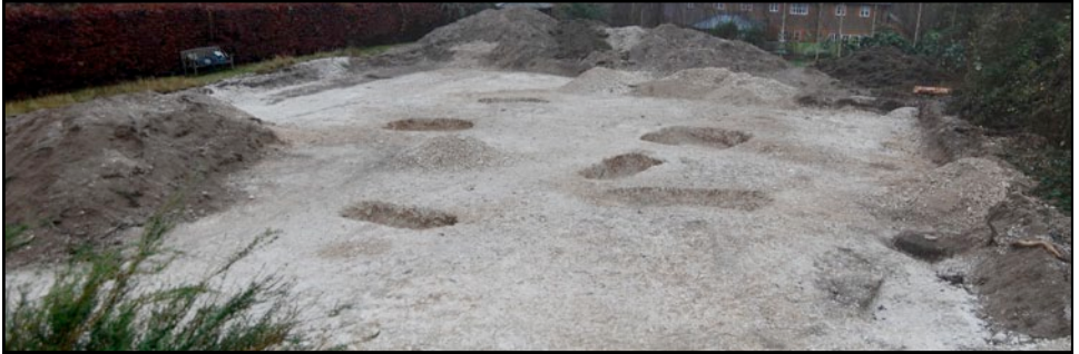
The excavated area at 12 Guildown Avenue
