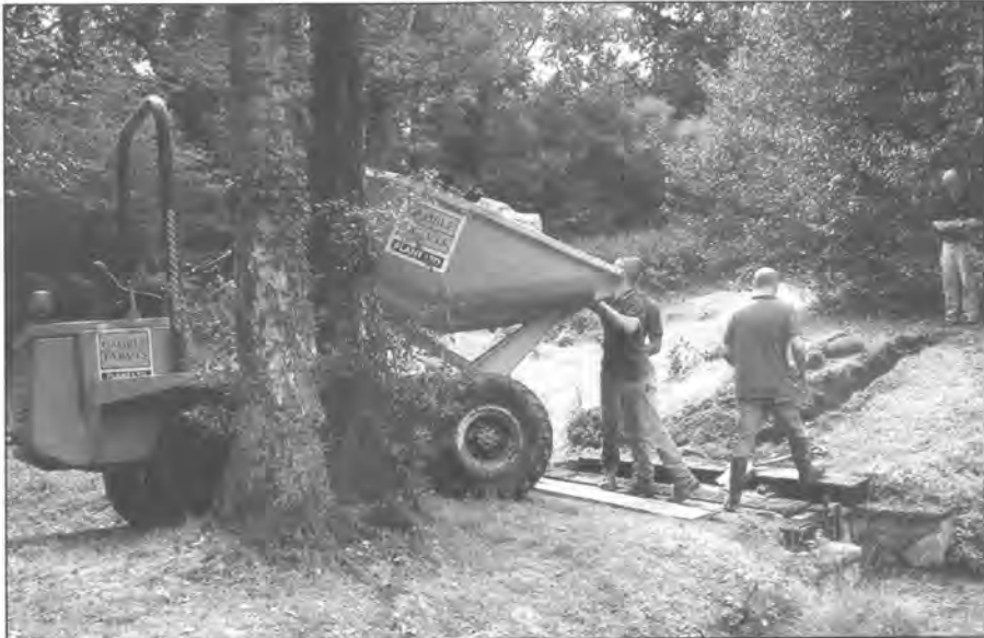
South Park Moat: filling the trench with bentonite.
