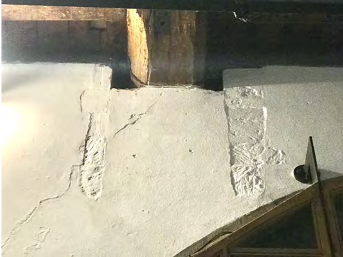
Fig 4 Bletchingley, detail of northern blocked opening as seen from within the tower. The uppermost block on the right-hand side looks to make a right-angle turn rather than commence a splay angle (note what appear to be vertically-laid bricks on the opposite side).
