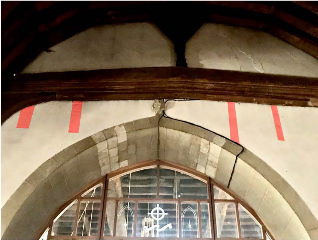
Fig 2 Bletchingley, view from the nave looking westwards; the jambs of the blocked openings are highlighted in red.
