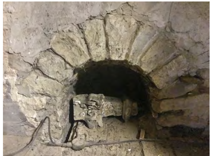
Fig 8 Bletchingley, reconstructed semicircular-headed opening in clock chamber east wall.
