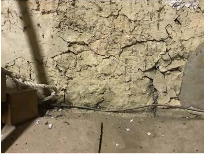
Fig 9 Bletchingley, possible blocked head of opening in clock chamber east wall.
