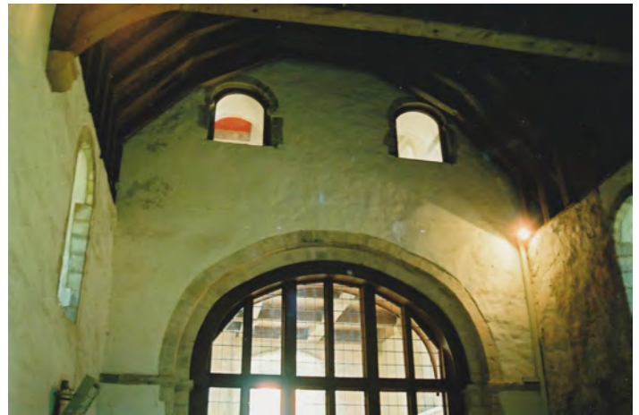
Fig 5 Brook, first floor openings viewed from the nave in 2007
