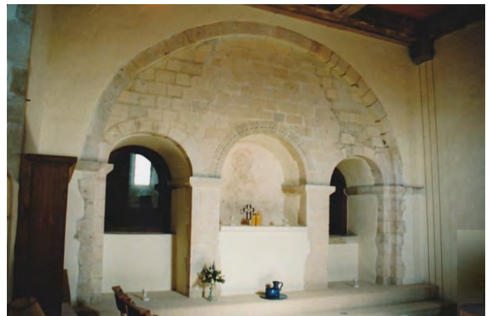
Fig 6 Brook, the east wall of the first-floor chamber in 2007. Note the regular ashlar construction of the jambs of the arches, superior in quality to what is visible at Bletchingley as shown most clearly in Fig 3.
