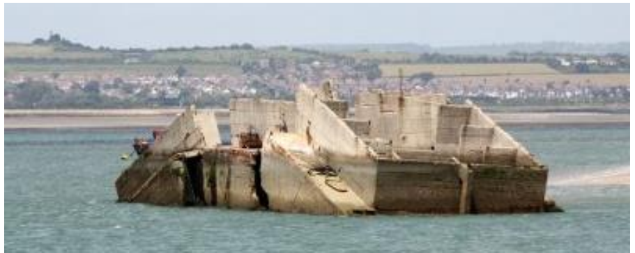
Broken Caisson in Langstone Harbour
