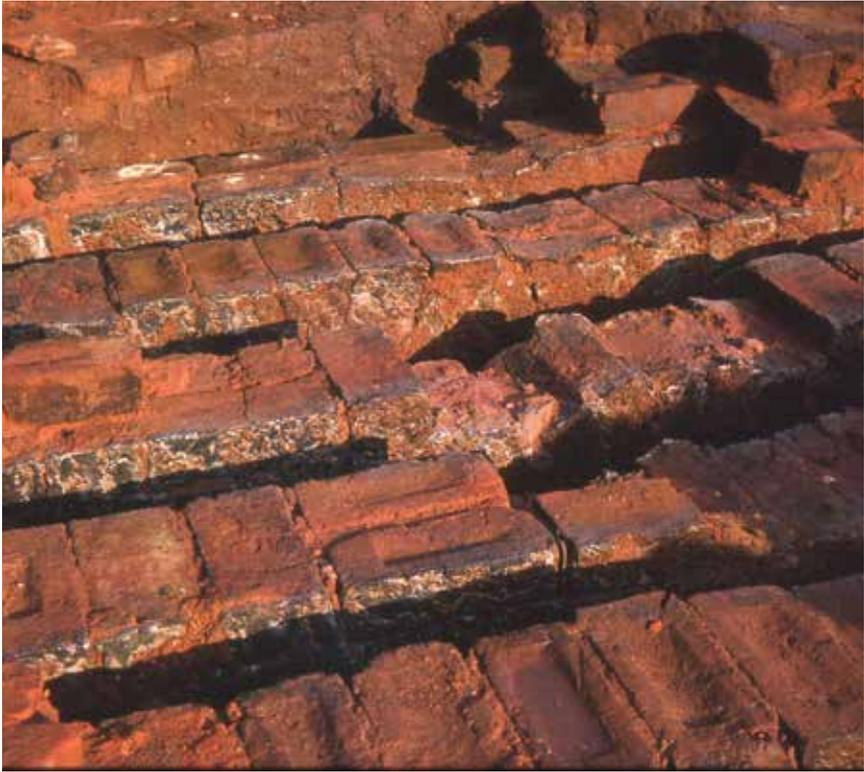
**Fig.5. Fire arches of the kiln. (Wardle.)**
