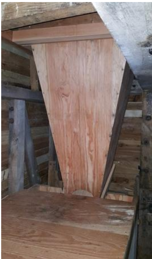
Feed hopper and top of bolter at stone floor level
