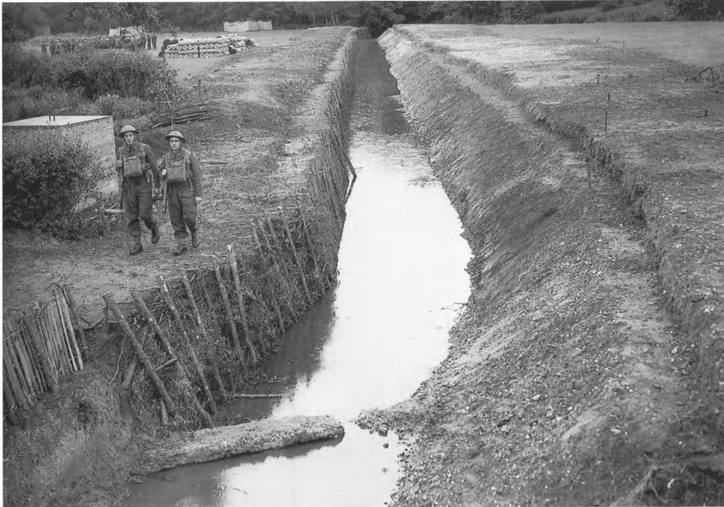
Fig 18.6 Patrolling a dry anti-tank ditch (containing some rain-water) behind Barfield School, Runfold, Farnham (SU 868 472). This is an example of a 'one-way' ditch with one vertical and one sloping side. The recommended dimensions were 15ft (4.6m) wide at the top, 6½ft (2m) wide at the bottom and 5ft (1.5m) deep (Wills 1985, 40), which appear to have been well-adhered to in this case. Photograph courtesy of the Imperial War Museum, London (H2473)
