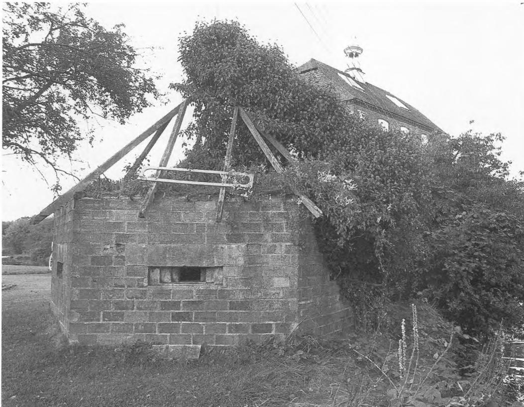
Fig 18.2 Photograph, taken in 1989, of an hexagonal pillbox on the GHQ line alongside the river Wey at Elstead Mill. It has rifle loopholes and the remains of camouflage which made it appear to be a summer-house. Photograph by Chris Shepherd
