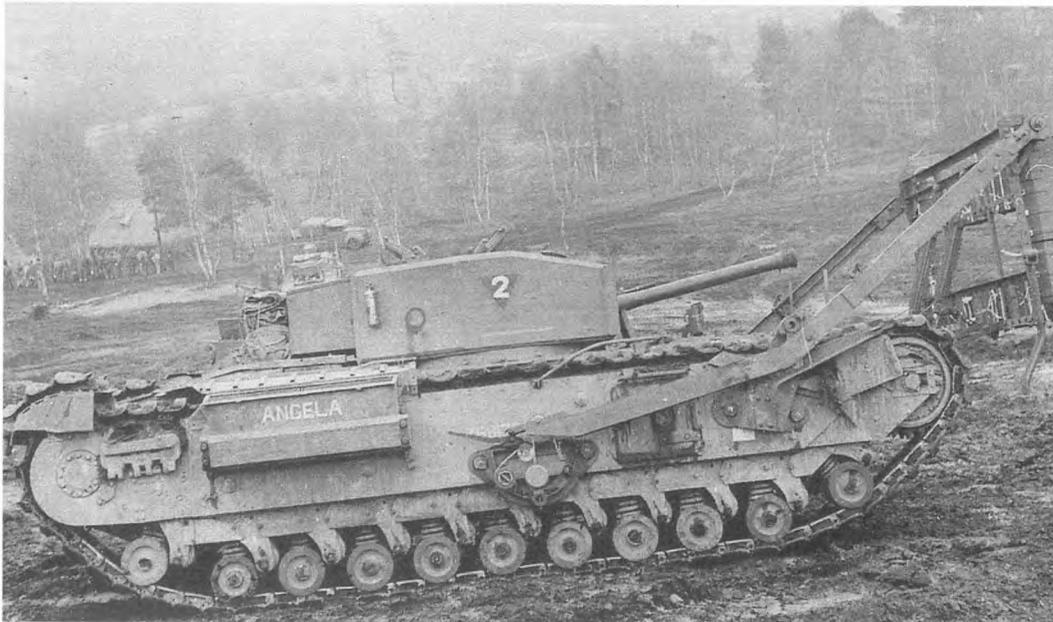
Fig 18.8 Churchill tank equipped with a steel frame capable of placing demolition charges at heights of up to about 4m. Courtesy of the Tank Museum, Bovington, Dorset
