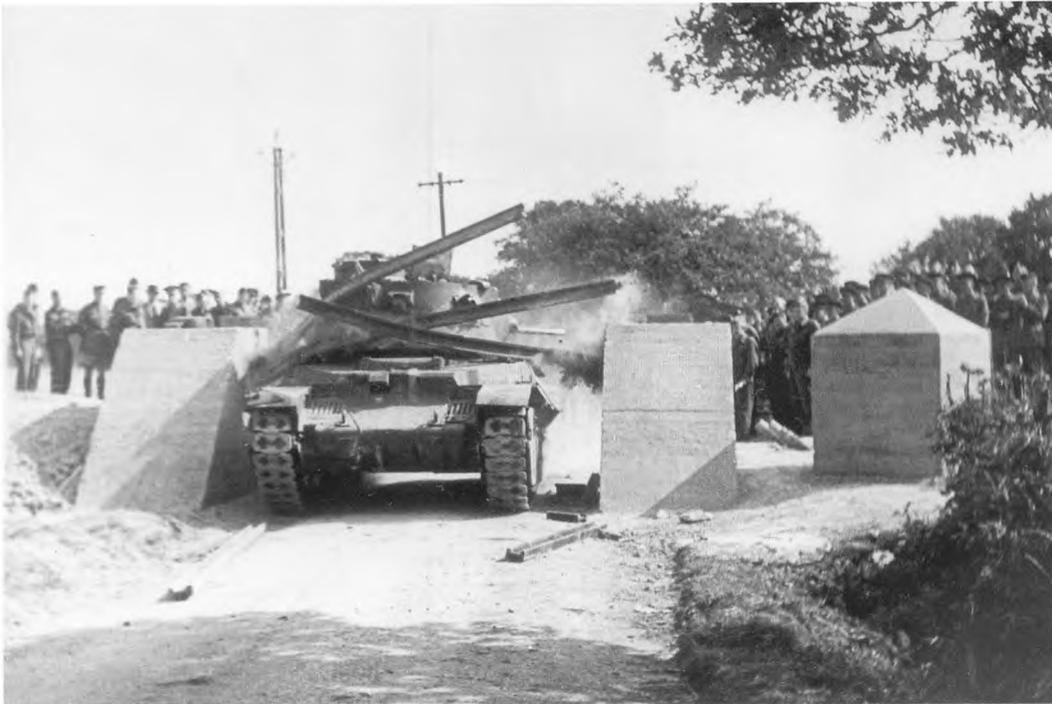
Fig 18.4 An anti-tank obstacle, consisting of concrete blocks and steel girders, being tested somewhere in Surrey. Courtesy of The National Archives (PRO: WO 179/15)
