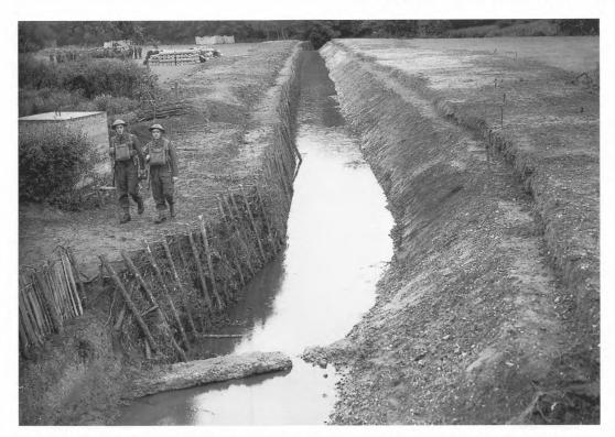
Fig 18.6 Patrolling a dry anti-tank ditch (containing some rain-water) behind Barfield School, Runfold, Farnham (SU 868 472). This is an example of a 'one-way' ditch with one vertical and one sloping side. The recommended dimensions were 15ft (4.6m) wide at the top, 61/2ft (2m) wide at the bottom and 5ft (1.5m) deep (Wills 1985, 40), which appear to have been well-adhered to in this case. Photograph courtesy of the Imperial War Museum, London (H2473)
