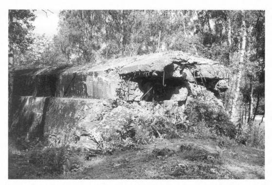
Fig 18.9 Part of the replica Atlantic Wall on Hankley Common, between Elstead and Tilford, showing one of the breaches created by explosives deposited against it by a Churchill tank in 1943. Note the broken iron reinforcement bars and the defensive platform on the near side of the wall. Photograph by Glenys Crocker
