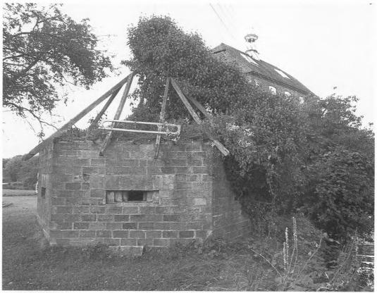
Fig 18.2 Photograph, taken in 1989, of an hexagonal pillbox on the GHQ line alongside the river Wey at Elstead Mill. It has rifle loopholes and the remains of camouflage which made it appear to be a summer-house. Photograph by Chris Shepheard
