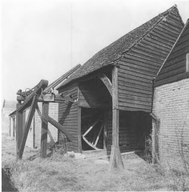
Fig 15.2 Treadwheel crane on the Wey Navigation at Guildford. One of the few treadwheel-operated cranes surviving in Britain, now located on the redeveloped riverside, close to its original site on Guildford Wharf. Probably dating from the late 17th century, it was restored by Guildford Borough Council for the National Trust in 1971. Similar cranes used to exist at Stonebridge Wharf, Shalford, and Godalming; Guildford Museum (G9431A)
