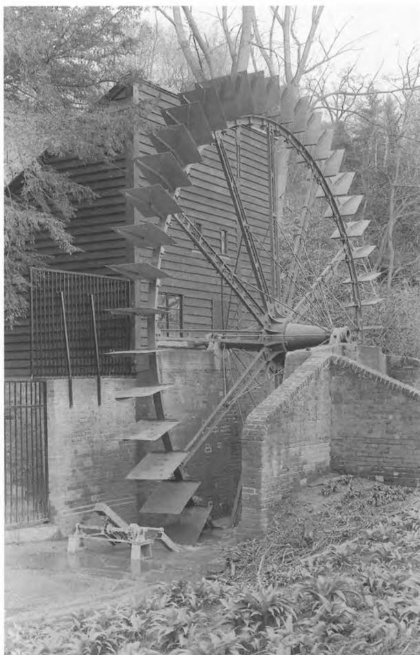
Fig 15.4 Water-wheel in Painshill Park. This 9m-diameter wheel was made by Bramah and Son in the 1830s to pump water to an ornamental lake and was restored in 1988. Technology played an essential role in many designed landscapes of the 18th and 19th centuries. Photograph by Jack Chinn, courtesy of Painshill Park Trust
