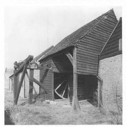
Fig 15.2 Treadwheel crane on the Wev Navigation at Guildford. One of the few treadwheel-operated cranes surviving in Britain, now located on the redeveloped riverside, close to its original site on Guildford Wharf. Probably dating from the late 17th century, it was restored by Guildford Borough Council for the National Trust in 1971. Similar cranes used to exist at Stonebridge Wharf, Shalford, and Godalming. Guildford Museum (G9431A)
