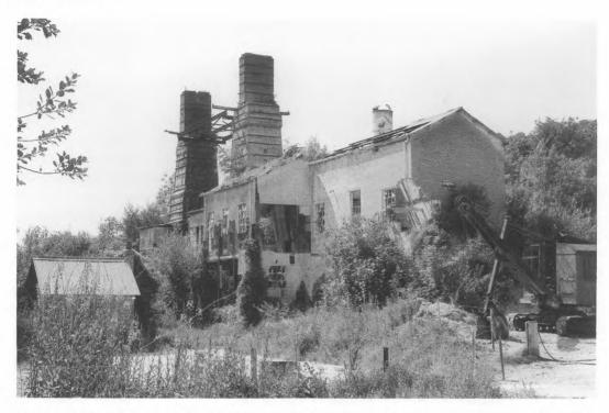
Fig 15.5 Betchworth limekilns. These kilns form part of the industrial landscape of the chalkpits and limeworks on the North Downs. The Betchworth site was worked from 1865 to 1934 by the Dorking Greystone Lime Company and these rare Dietzsch kilns were added in the 1890s to convert chalk into quicklime. The 1924 hydrator for converting the quicklime to slaked lime, seen to the right of the kilns, went out of use in 1956 and has since been demolished. Photograph by Paul Sowan
