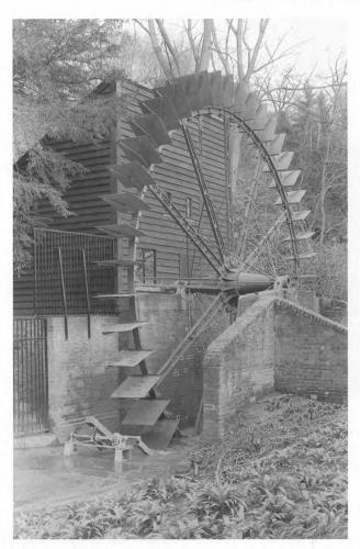
Fig 15.4 Water-wheel in Painshill Park. This 9m-diameter wheel was made by Bramah and Son in the 1830s to pump water to an ornamental lake and was restored in 1988. Technology played an essential role in many designed landscapes of the 18th and 19th centuries. Photograph by Jack Chinn, courtesy of Painshill Park Trust
