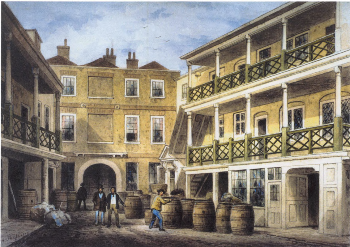
Fig 14.1 The yard of the Bell Inn, Aldersgate, drawn by T H Shepherd in 1857. Though this is a central London example, it shows the variety of building components to be sought when looking for inns at smaller towns: galleries, a variety of window forms, and a mixture of brick and timber walls. Guildhall Library (79)
