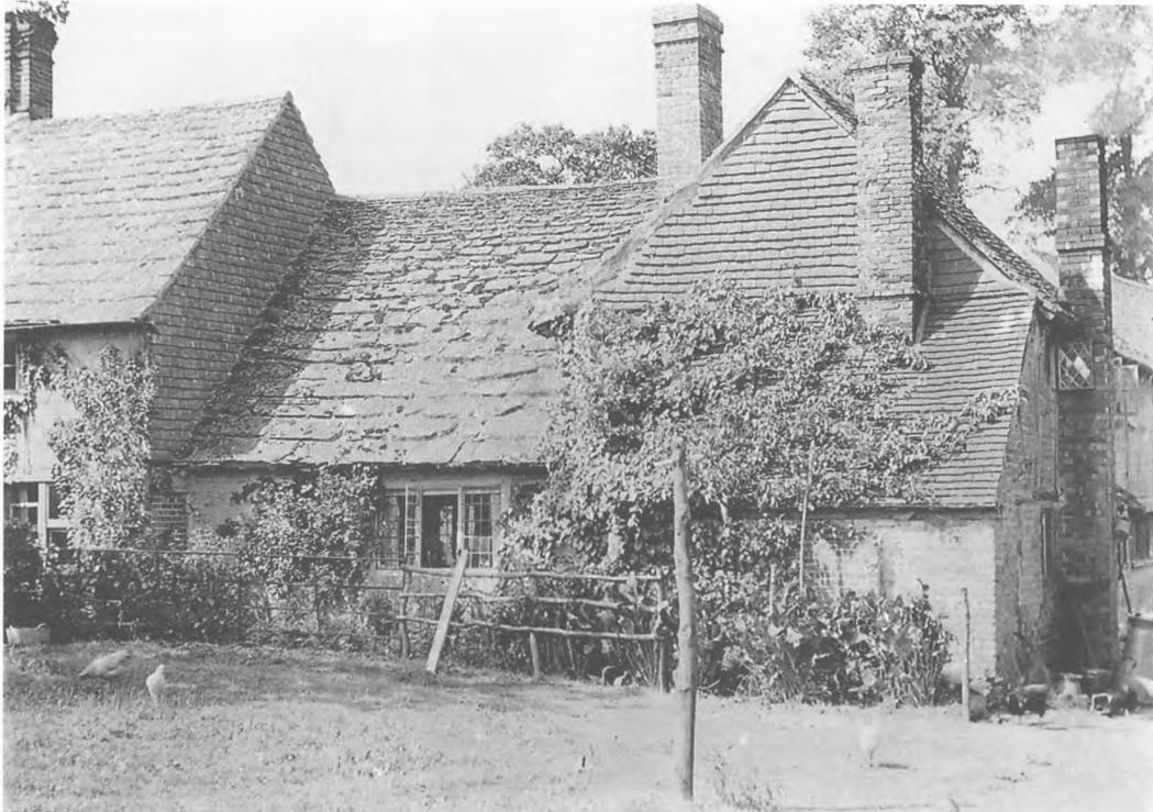
Fig 11.2 Aldhurst Farm from the rear. This shows the smoke-bay range to the left, the end elevation of the detached kitchen from Tepehams on the right, and the central linking bay. Reproduced by permission of Surrey History Service: Surrey Photographic Record 2873. Copyright of Surrey History Service
