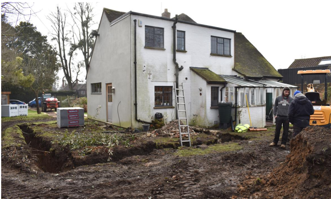
Pennys, 88B West Street, showing the north-east extension footing trench.
