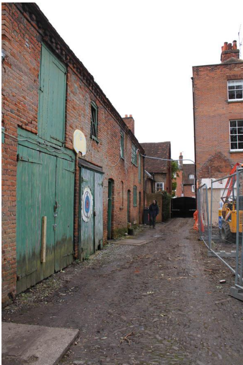
Fig 3 Cobbled access drive, looking towards Castle Street.
