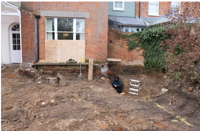
Fig 5 Open footing trench.
