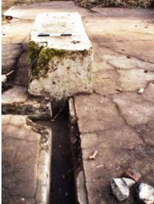
One of the two gullies
