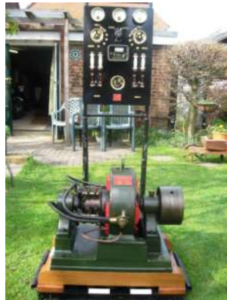
Example of control board
