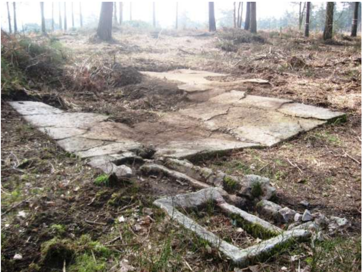
Concrete base showing catchment pit
