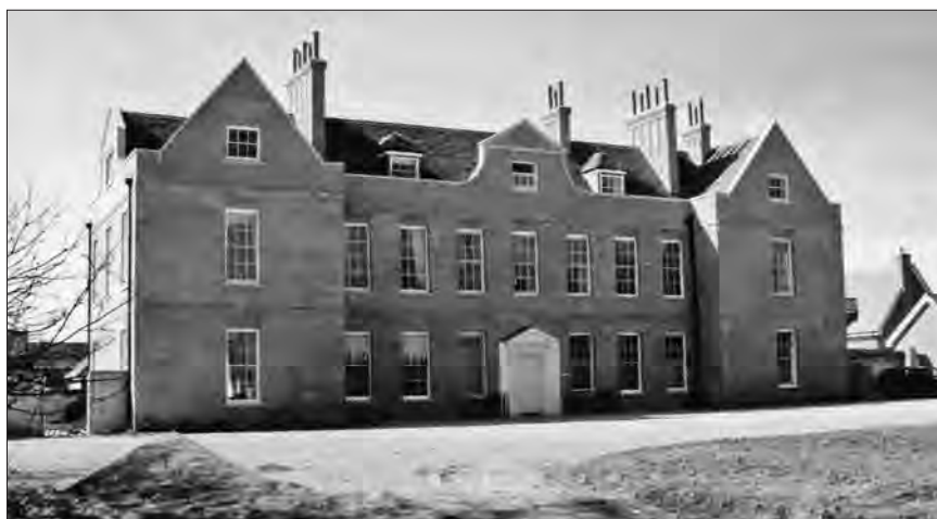
Figure 4 East façade of Henley Park Mansion after restoration in 1999 (Pat Ashworth)
