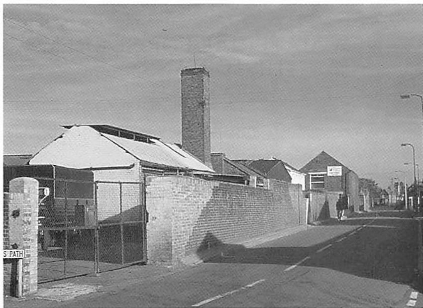
Fig. 15. The works of George Purdom & Co. in Church Road, Mitcham, in 1974.
