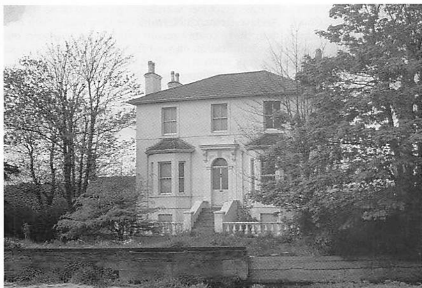
Fig. 16. Paul Addington's Villa, Phipps Bridge, in 1972.
