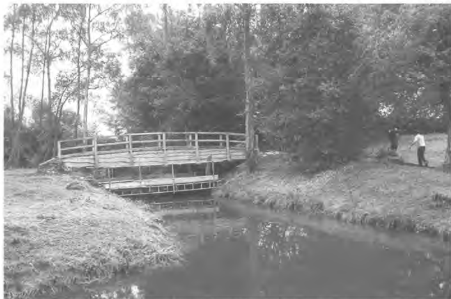
South Park Moat: Bridge under repair with temporary scaffolding in place
