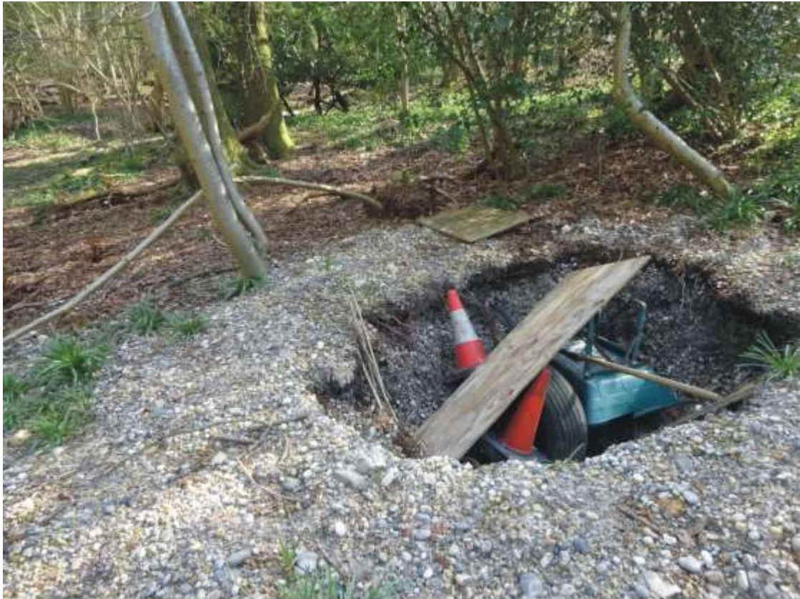
Figure 19 Gravel exposed during modern works
