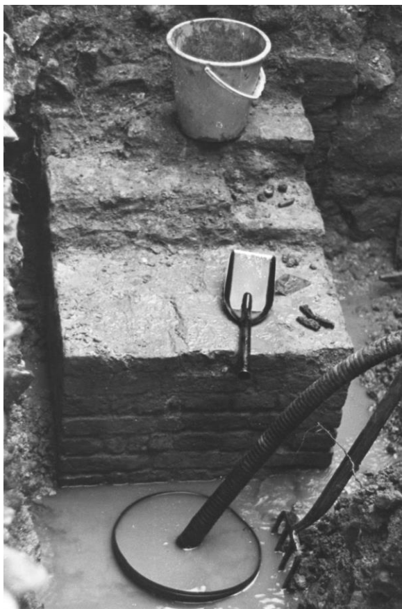
Fig 11 Guildford Park Manor. Photograph of the 'Tudor' brick abutment or pier projecting from the revetment wall at the west end of A and B*, taken while water was being pumped away.
