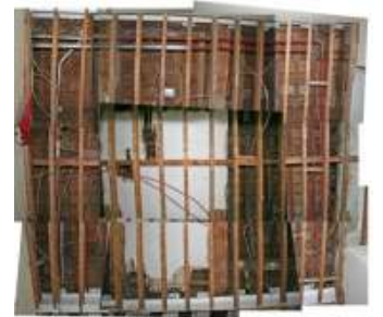
FC44 Rooms A & B ceiling
