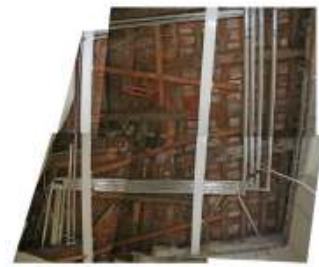
FC30 Room C ceiling
