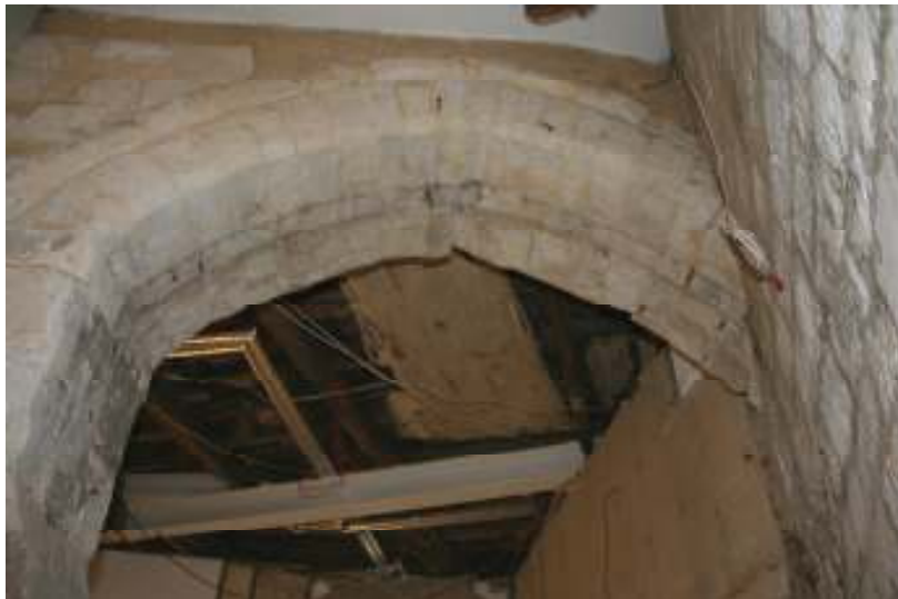
Archway exposed during works
