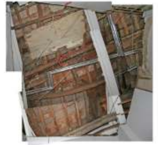
FC24 Room D ceiling
